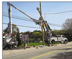
Repair work continues Tuesday after a car crashed into a pole.
